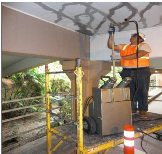
(c) Epoxy pressure injection to slab.
