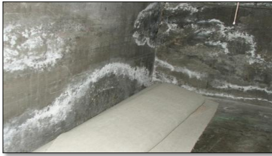
(c) Efflorescence in concrete
