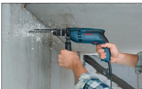
(a) Drilling of concrete element
