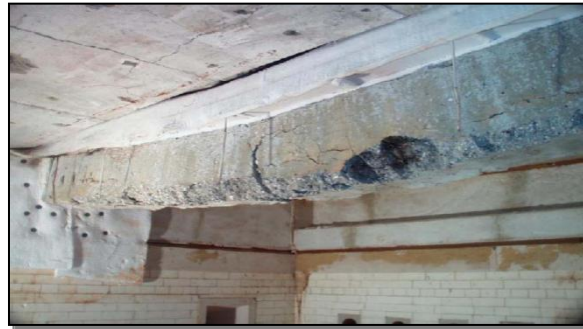
Figure 2: Shear Crack on Beam
