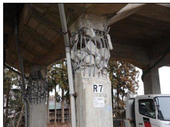
(b) Crushing of Column.
