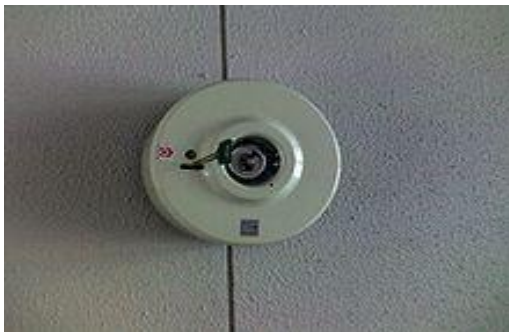
A small emergency light
