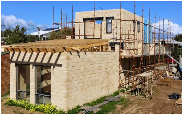
Fig. 2.31: Application of Timbercrete in Building
