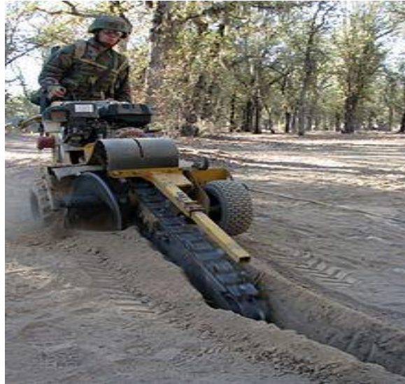
Fig. 3.19: Portable Assault Trencher Machine in Operation
