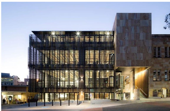
Fig. 2.27: Queensland's University GCI Building With 3 Suspended Floors Made From Structural Geo-polymer Concrete
