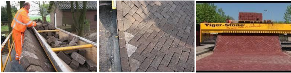
Fig. 5.9: Working of Road Printers
