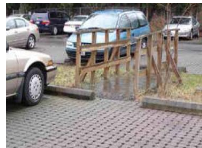
Fig. 2.19: Use of Pavers As Porous Pavement
