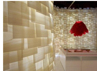
Fig 2.8: Walls with Translucent Wood
