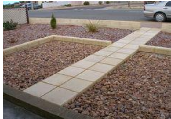
Fig. 2.32: Timbercrete as Paver
