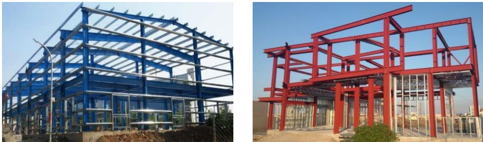
Fig. 5.4: Pre-engineered Steel building and Conventional Steel Building
