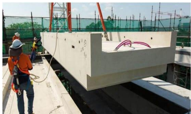
Fig. 2.28: One of The 33 Precast Slag/Fly Ash-Based Geo-polymer Concrete Floor Parts
