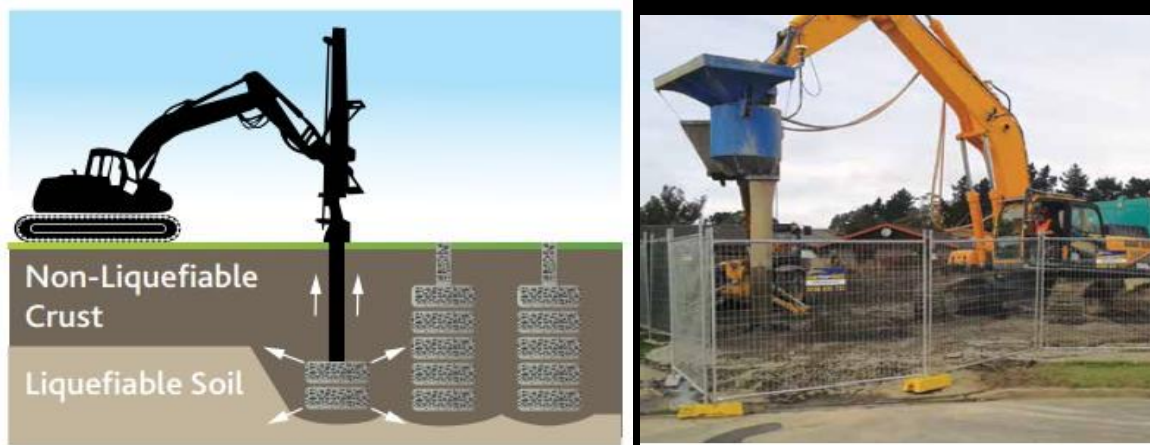
Fig. 5.16: Construction of stone column
