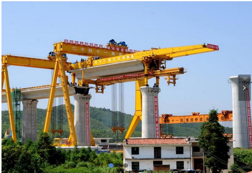
Fig. 3.26: Bridge Girder Launcher
