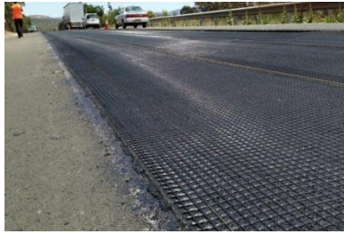
Fig. 2.13: Use in Road Construction
