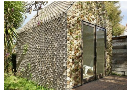
Fig. 2.11: 3D Printed Tiles as Walls Exteriors
